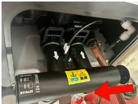
Bypass Mode: Piston Closed Image 15
