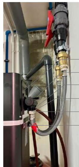
All Water Connections Completed Image 18
