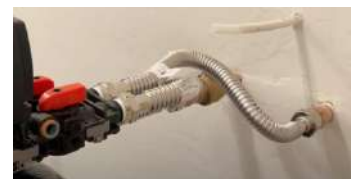
Inlet & Outlet Pipes Connected to the Bypass Valve on Softener Image 3
