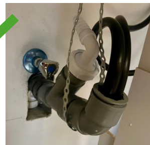
Double-Waste Outlet for Washing Machine + Waste & Overflow for Softener Image 14
