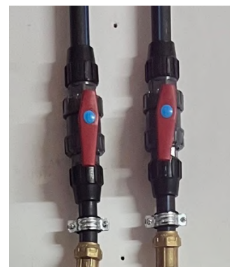
Inlet & Outlet Valves Fully Open Image 23
