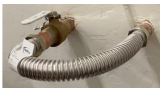
Softener Loop with Isolator Valve at the Inlet Image 1
