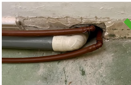
Waste & Overflow Pipes in Floor Drainage Image 13
