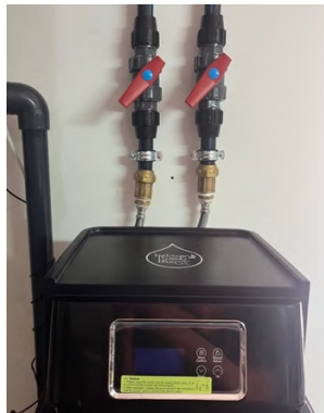
Inlet & Outlet Valves 1/2 Open Image 22
