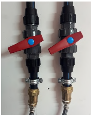
Inlet & Outlet Valves 1/3 Open Image 21
