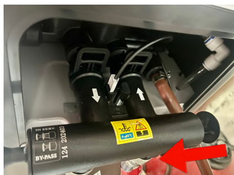
Bypass Mode: Piston Closed Image 15
