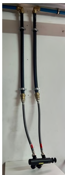
Mains Inlet, Outlet & Bypass Valve Connected Image 17
